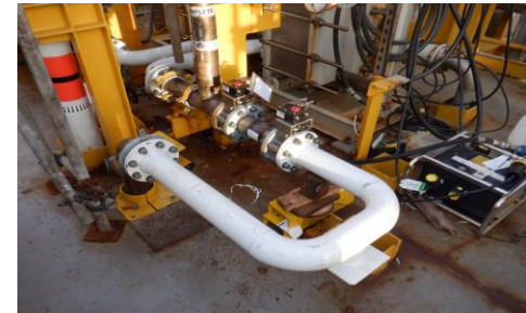
FPF1 – Pipework replacement
