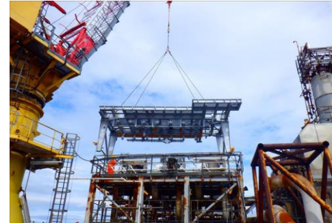
Captain – New deck installation
