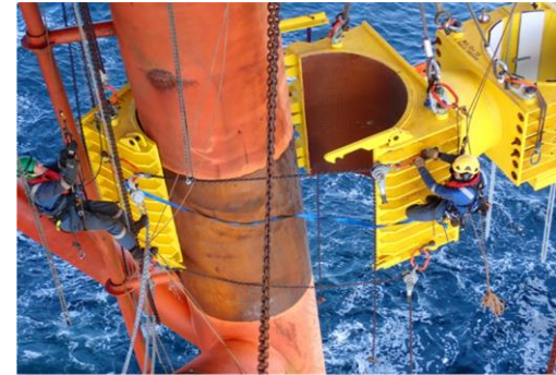
Captain EORII - Riser caisson clamp installation
