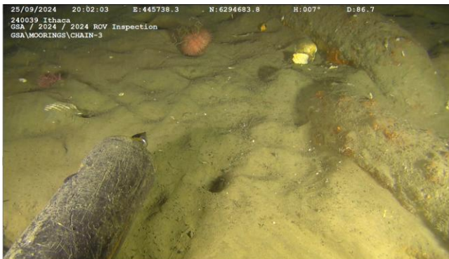
Figure A.3: Photos of seabed around FPF-1 mooring chain 2 and anchor piles
